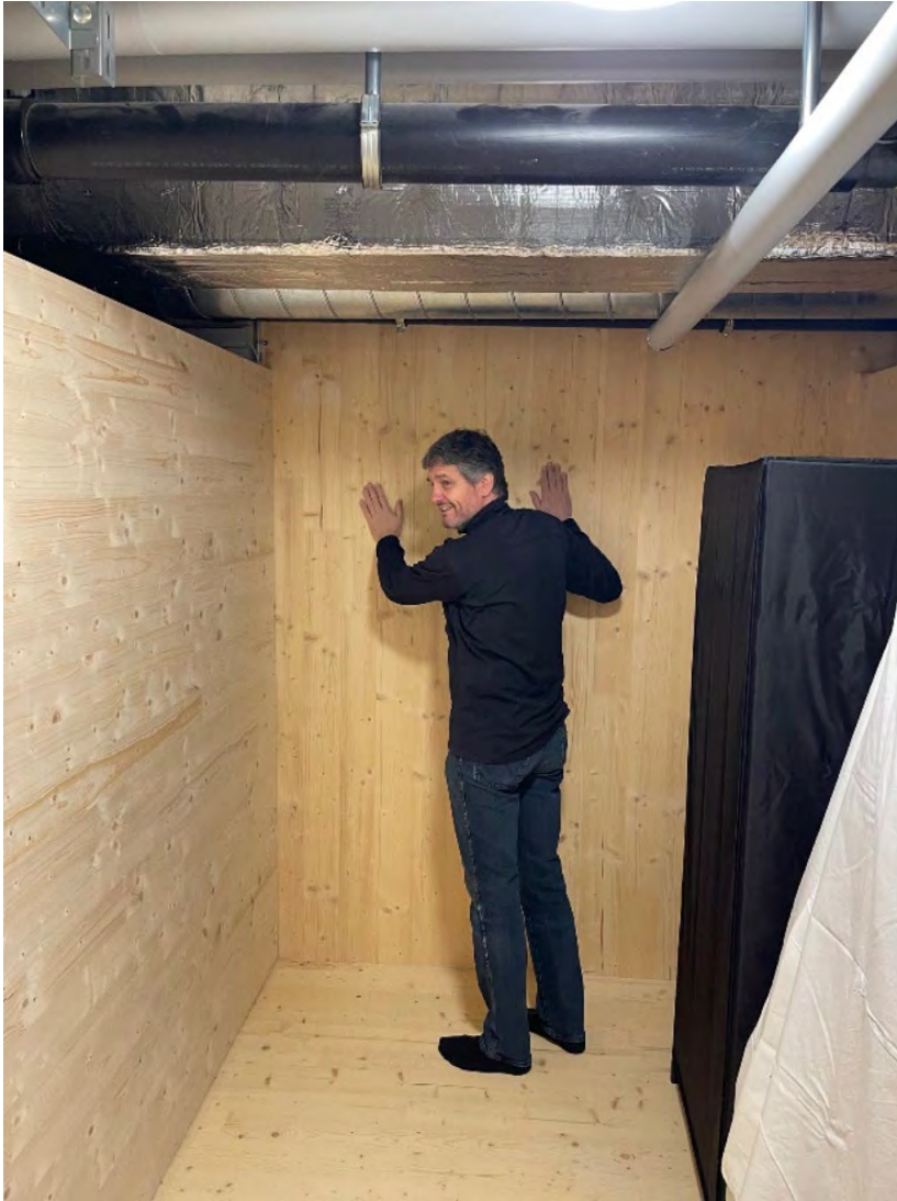
Figure 7 - Exposed Interior Surface of the CLT Foundation Wall, Residential Project in Thun, Switzerland.
